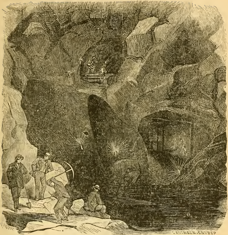
IN THE WEST JORDAN MINE.
